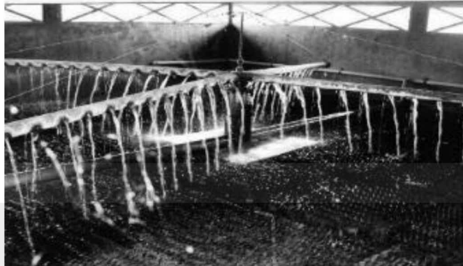
Figure 6. Trickling filter system installed at Taman Indah Permai, Kota Kinabalu
