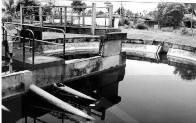
Figure 4. Oxidation ditch installed at King Fisher Park, Kota Kinabalu
